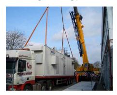
The hospital also benefited from a new waste heat boiler which required the original boiler house façade to be removed to allow the installation and integration to the existing system.
