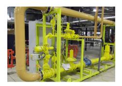
Biogas is produced on site via Arla Food's anaerobic digester, which treats the sites influent. There is sufficient biogas to produce approximately 400kWe, which represents roughly 10% of the total CHP load (4MWe).
