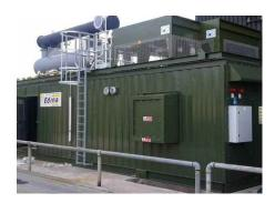
Additional acoustic panels were fitted externally to attenuate the transfer of noise to neighbouring buildings and the CHP container was built, coloured and installed to blend in with its surroundings and to be as unobtrusive as possible.
