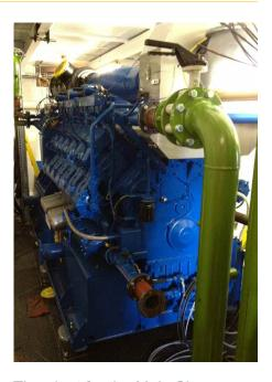
The plant for the Main Site was containerised in an attenuated, acoustic enclosure at Edina's manufacturing facility, based in Lisburn, Northern Ireland and included full heat recovery from the engine jacket water, lube oil, intercooler and exhaust gases.
