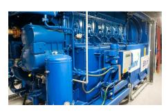
The scope also included the construction of a purpose built energy centre which houses the TCG 2032 engine, associated ancillary plant and separate waste heat steam boiler room.
