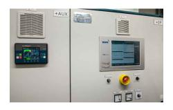
The CHP plant will be remotely monitored 24/7 by Edina via its SCADA (Supervisory Control and Data Acquisition) systems, which will automatically detect and alert Edina's service desk of any issues on-site.
