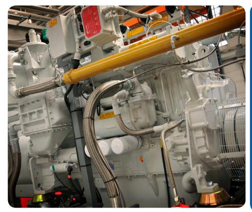
The data centre solution accommodates a 425kWe trigeneration unit that uses an efficient Perkins engine. This unit accommodates the no-break provision promise to ensure island mode is possible.
